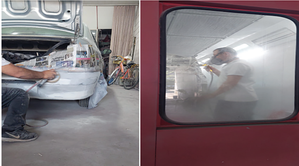
Image 1. Vehicle preparation and painting process in the paint booth
